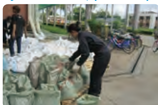
Building a sandbag dike for flood protection
