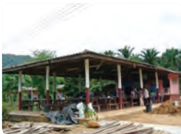
Canteen before replacement
