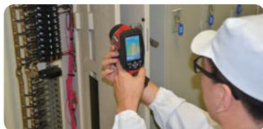
Early detection of power distribution panel problems using thermography
