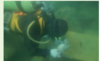
On-site monitoring of “organic concrete”
