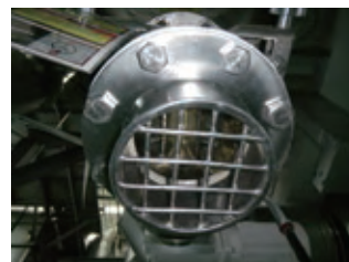
Wire grille installed
