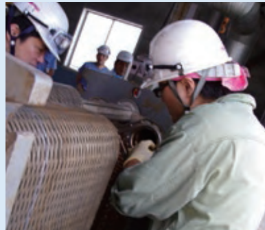
Ensuring stable production by taking apart a heat exchanger and washing each section by hand
