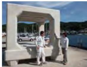
An artificial fish reef made from the Environment Vitalizing Concrete was installed on the sea bottom, which was eight meters deep, about one kilometer off the port of Ito in Shizuoka Prefecture.
