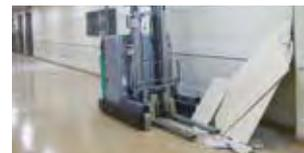
Production floor: Water leaks, distortion in walls and ceiling, walls damaged
