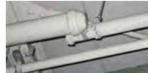
Machine room: Pipes damaged, metal fittings damaged and fallen
